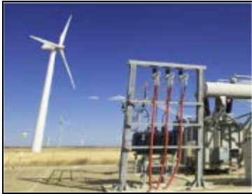
Grid Connection of RES Wind, Solar & more Energy & Battery Storage
